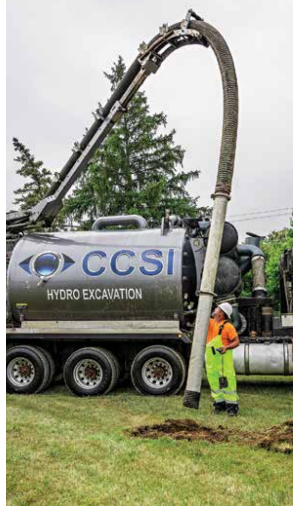
Operator Steve Nichols moves the boom for more potholing work.
