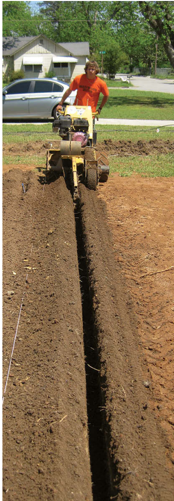
Lexington Belyeu guides the Vermeer trencher through heavy Georgia soil.
