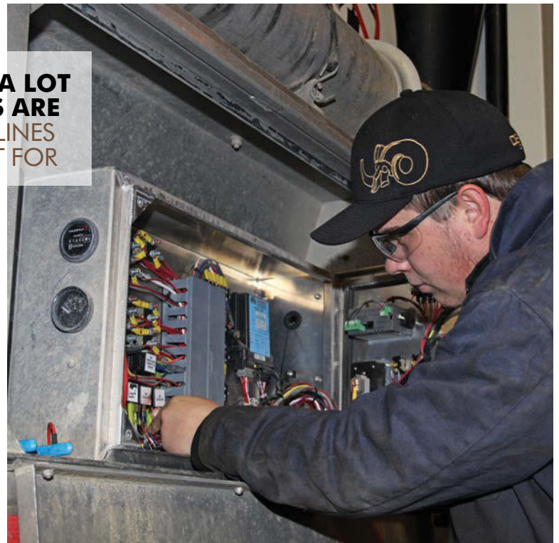
Marcus Baker, mechanic, works on one of the company’s hydroexcavators at its shop in Mountain View.
