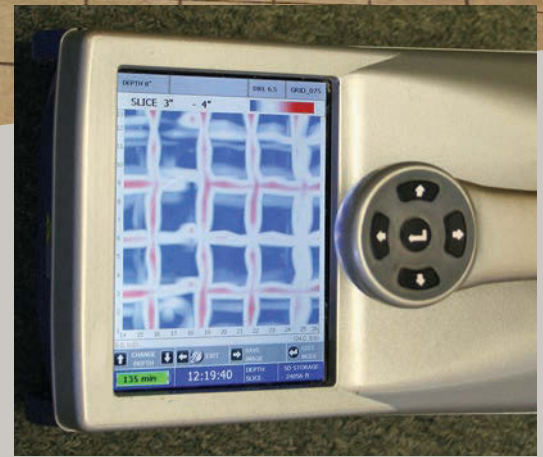
TOP PHOTO: The GSSI StructureScan Mini HR (High-Res) being guided by laser along a pre-drawn grid on the floor. INSET: The screen displays rebar beneath the carpeted concrete slab floor in Pegasus headquarters.
