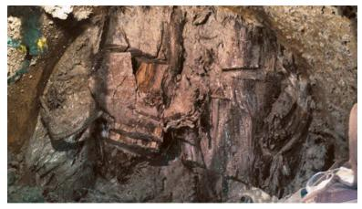
Crew must remove a 5-foot-diameter tree stump buried during original construction of railway substructure.
