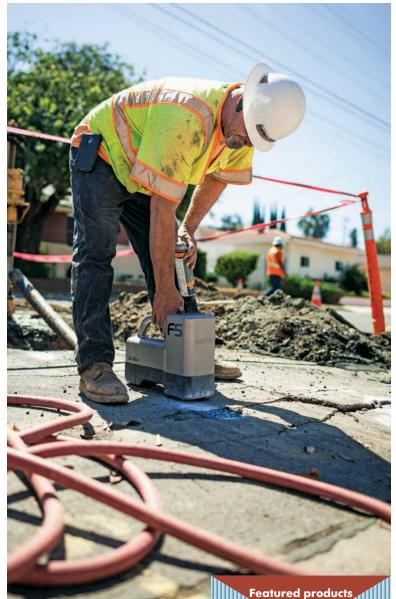
California Boring's Todd Minkey uses a Digital Control Incorporated DigiTrak F5 to help guide the directional drill toward the access pit.
