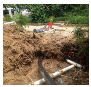
The 6- by 6- by 5-foot-deep entry pit was 6 feet upstream from the sauare stormwater vault with two 36-inch concrete drains.
