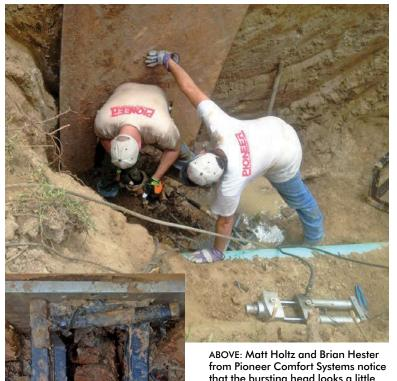
that the bursting head looks a little strange as it emerges through the resistance plate. A 4-inch cast iron check valve is wrapped around the head. LEFT: The check valve is pulled through a 4-inch clay tile lateral with a 45-degree elbow and a wye, then 60 feet to the pit.
