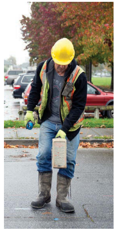
Crew member Paul Stancic paints a reference point while using a DigiTrak Mark III (Digital Control Inc.) to measure the location and angle of the horizontal directional drill's drill bit.
