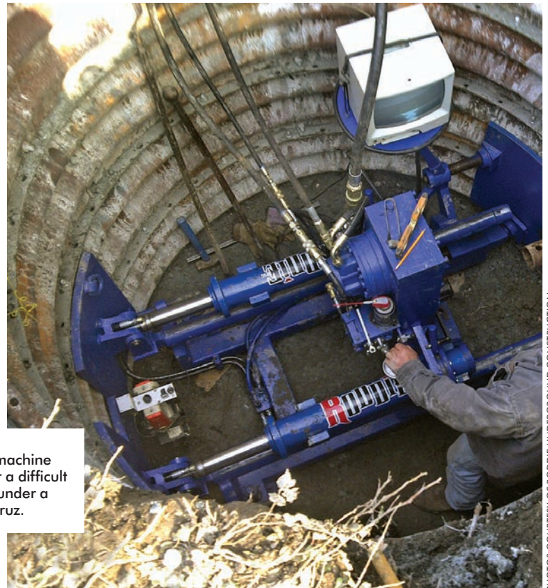
PHOTOS COURTESY OF RODDIE UNDERGROUND CONSTRUCTION
