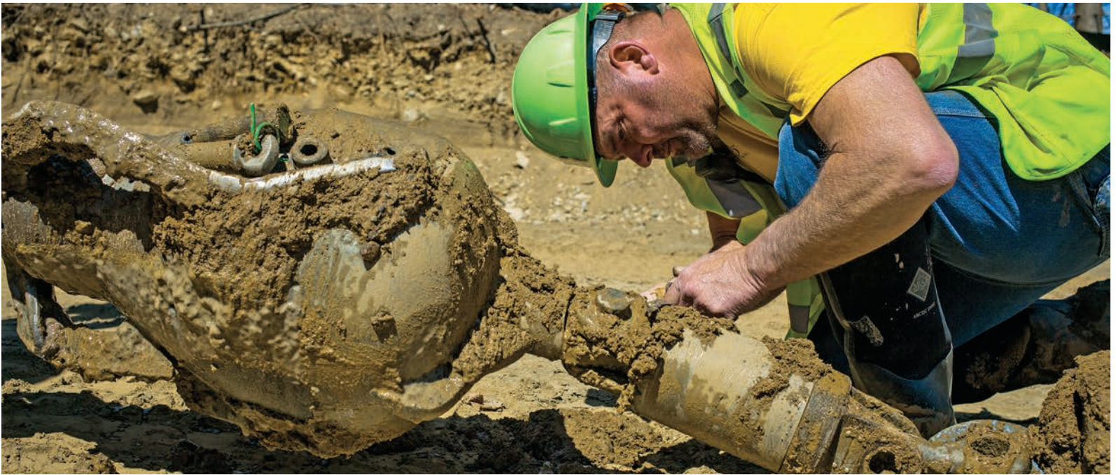
Drilling assistant Bill Martin disconnects the drill bit from the pipe being pulled through on a water main installation job.
