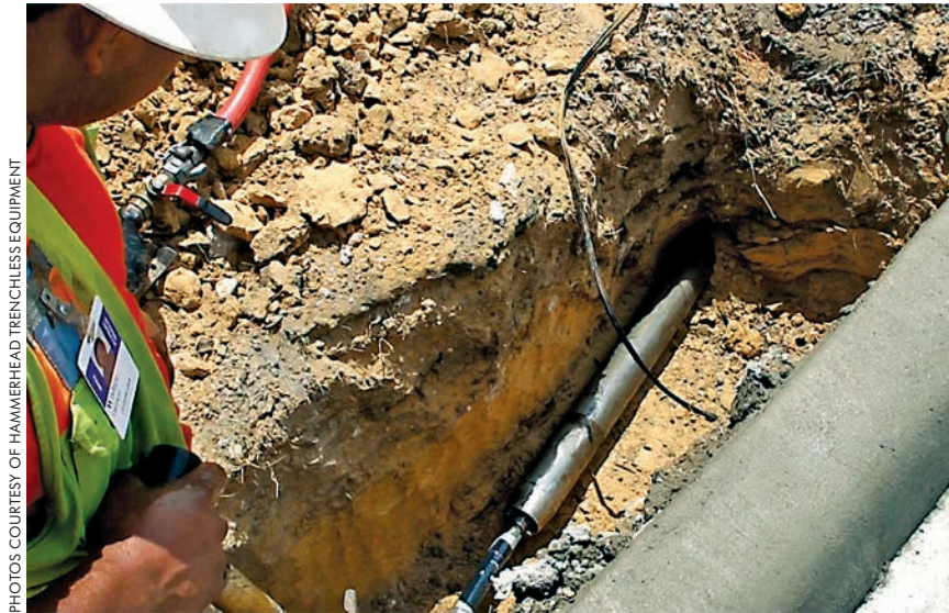
A contractor uses a piercing tool from HammerHead Trenchless Equipment on a job site. There are several piercing tools that can be selected from, depending on soil type and the job the contractor is doing.
