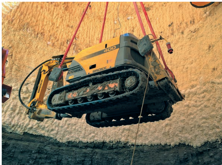
A crane slowly lowers the Brokk 400 machine into the shaft.
