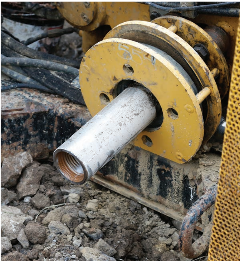
The directional drill without the tool attachment.
