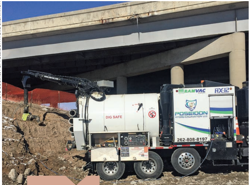
PHOTO COURTESY OF POSEIDON HYDRO EXCAVATION
