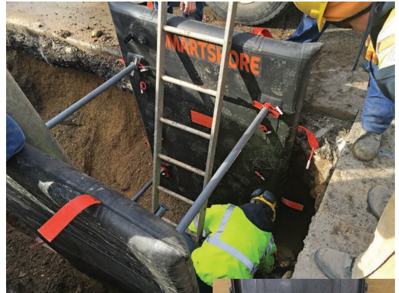
The Smartshore system sets up in as little as 10 minutes. With each section weighing only 29 pounds, it is easy for workers to transport and set in place.
