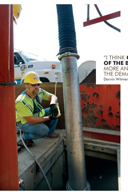
Dervin Witmer uses the hand controller to operate a Vactor 2100 hydroexcavator as the machine removes sand and stone from Kenneth Smith's Michigan Distribution Terminal.
