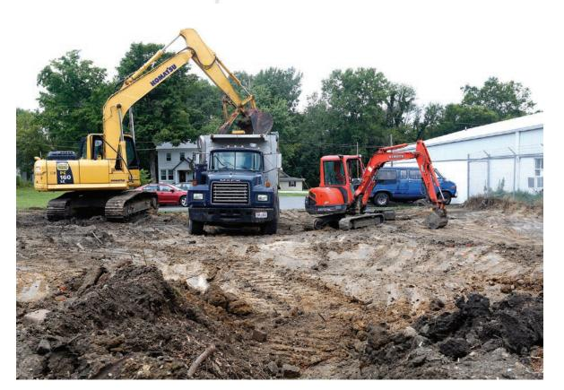
Jim Store uses a Komatsu PC160 to take the top soil down to the clay in order to build a parking lot.
