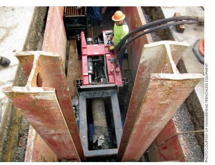
A HammerHead HB 125 static pipe bursting system offers contractors a machine that is versatile enough to replace a wide range of water, sewer and gas lines.
