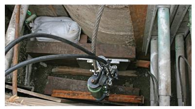
The manhole's cylindrical wall created a void to the left of the M50 ram that was filled with 6-inch timbers and two sandbags to make the resistance wall perpendicular to the pull force.
