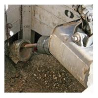
ABOVE: John Rafferty, director of marketing and technical support at TRIC Tools, attaches the pipe and head driver to the threaded cable end, LEFT: The backhoe bucket pushes down on the 8-inch HDPE pipe to assist the angle of entry.
