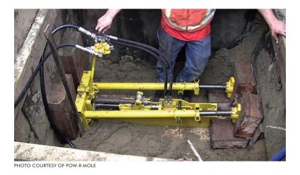
A contractor uses a Pow-r Mole PD-4 on a job site. The PD-4 can operate in a pit only 50 inches long or bigger and has a thrust force of 37,714 pounds at 3,000 psi and a maximum push rate of 9 feet per minute.
