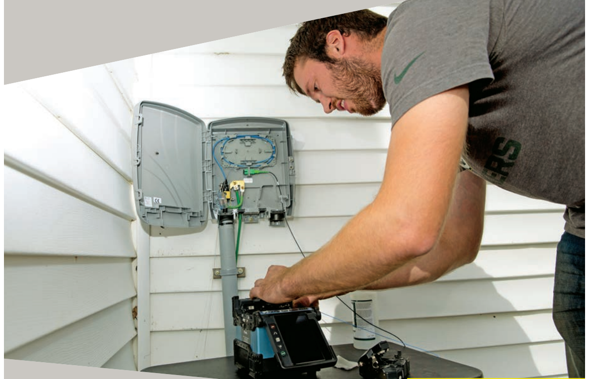
David Wilken splices fiber optic cable for a residential installation.
