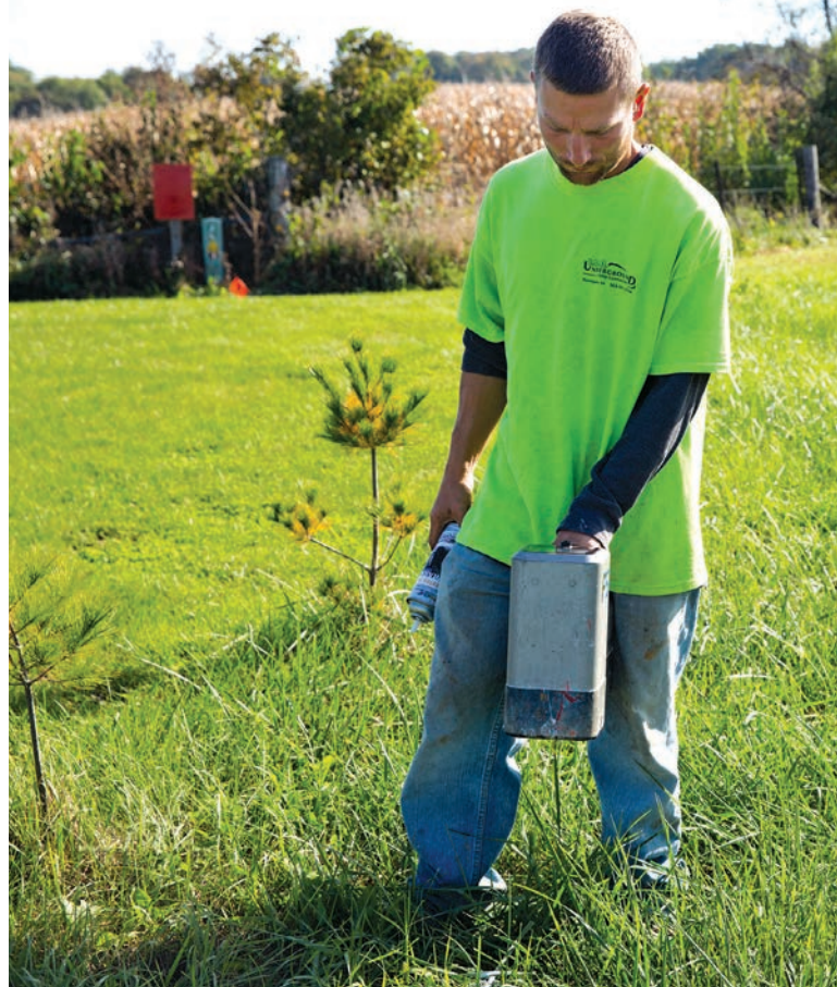
Nate Jurski uses a DigiTrak Model F5 (Digital Control) locating system to locate and direct the boring head on a job site.
