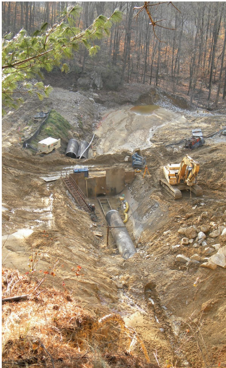
A view from the top of the cliff downstream at the jacking pit and HDPE pipe in its final position.
