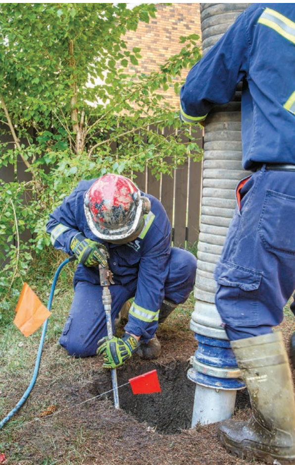
Ryan Dorchak (right) secures the hydroexcavator vacuum tube (Foremost) as Bryce Jeske uses the digging wand to break up dirt. (Roughneck Series safety gloves by Ringers Gloves.)
