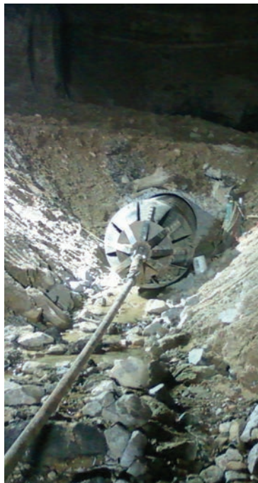
The pulling assembly emerges from the 66-inch casing into the spotlight. Once the pull began, it continued nonstop.
