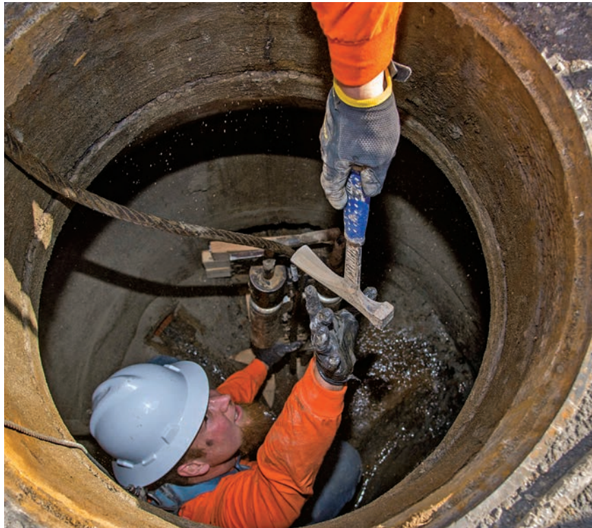
Technician Cody Pingree reaches for equipment as he waits for the bursting head to reach his location. The company was installing a new line from a home to the main sewer system.
