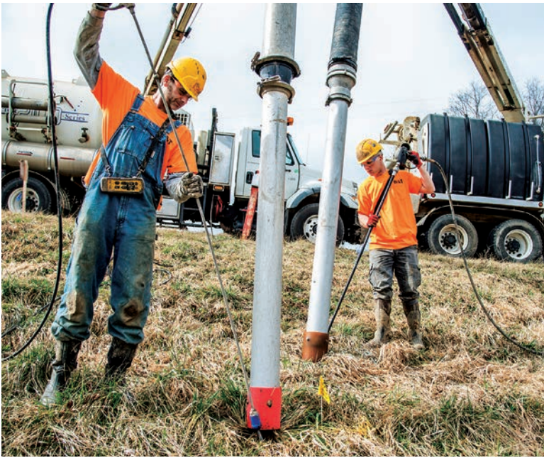
From left, technicians Abel English and Colby Boyer perform hydroexcavation work as part of the services offered by B&T Drainage (Vactor and Super Products).
