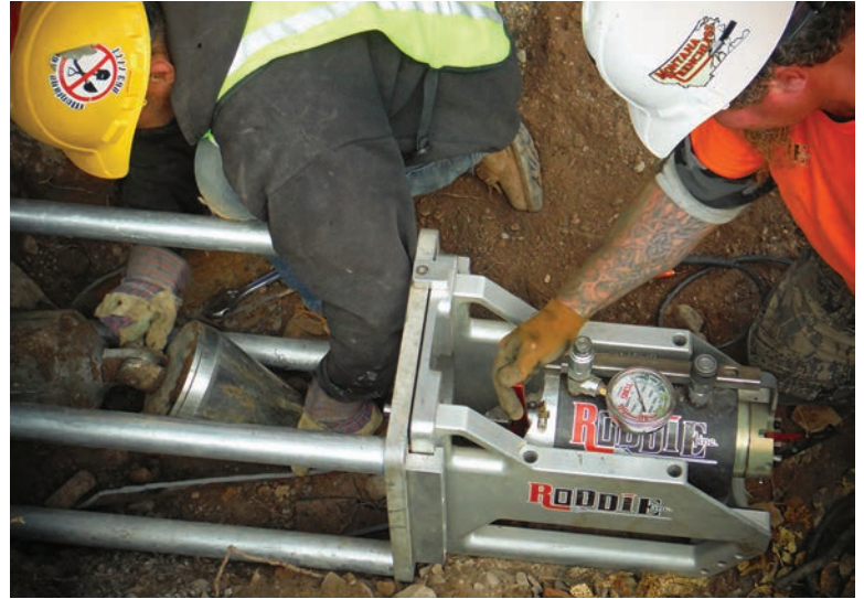
Adam Shappell (left) disconnects the 6-inch articulating bursting head while Jeff Hanson uses a wrench to remove the magnetic-assisted locking device connecting the head to the welded end of the 22 mm cable. Both workers are from Montana Trenchless.
