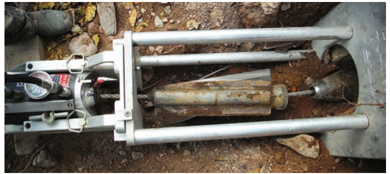
The custom-made 13- by 8.5-inch-wide slitting blade slips over the 22 mm cable, then seats against the nose of the 6-inch articulating bursting head.
