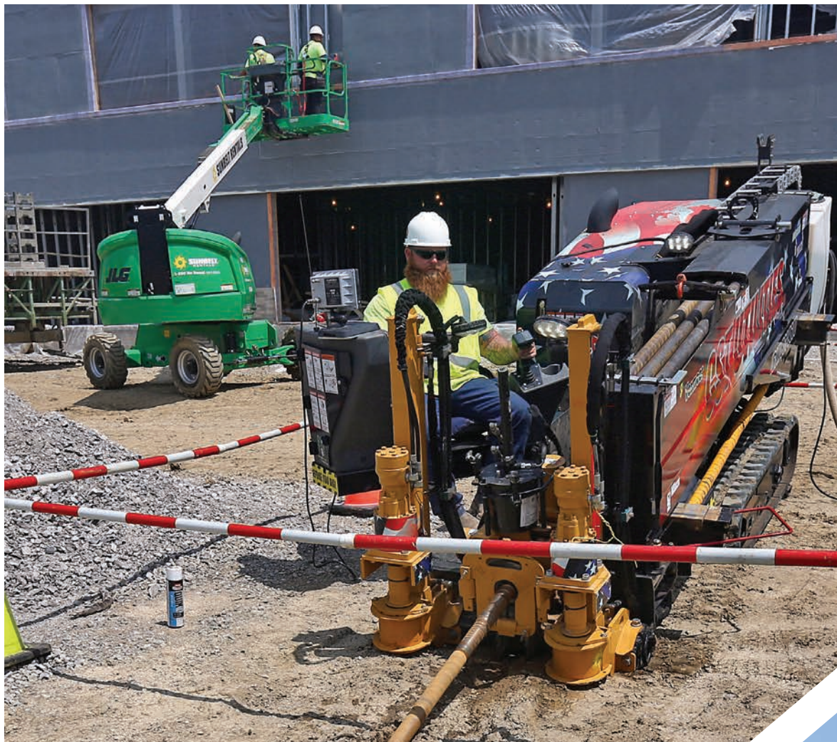
CST Utilities operator Nick Gilbert uses a Vermeer 20x22 directional drill while boring for new electrical lines for a new apartment building.
