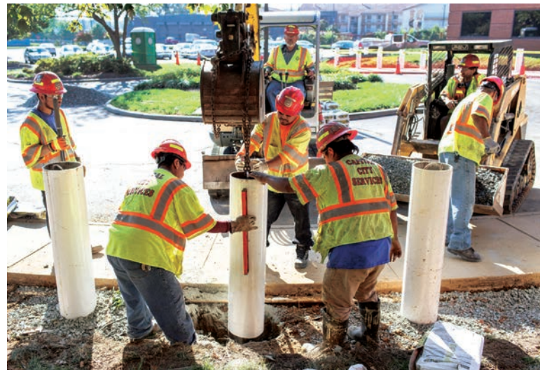
Capital City Services crew members (from left) Mario Flores, Pedro Xum, Reveriano Allendee and Jose Avila install bollards while company owner Wayne Norman holds the bollard in place with a compact excavator. David Conken sits nearby with a load of rock fill while Javier Sileo begins manual backfill.
