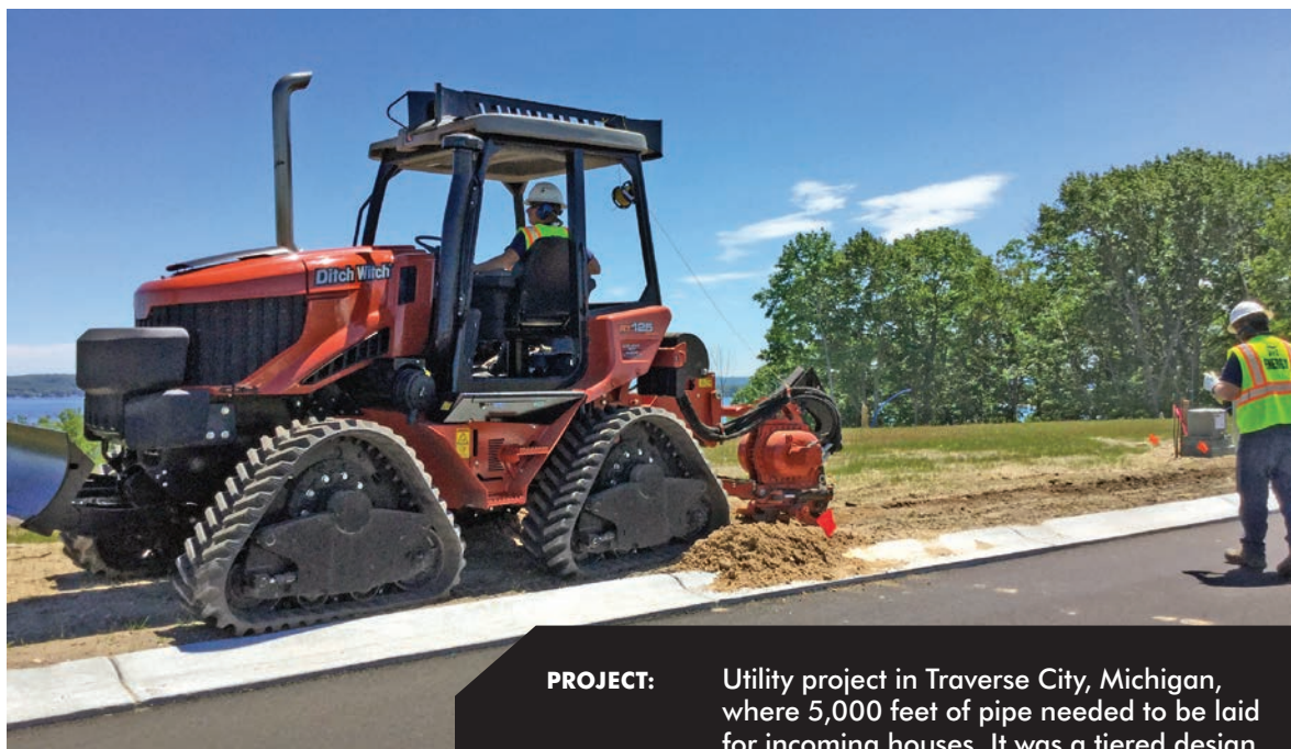
DTE Energy crew members use a Ditch Witch RT125 Quad utility tractor to dig a trench to install pipe on a housing project in Traverse City, Michigan. Over a single day, it put 3,000 feet of 2-inch pipe in the ground.
