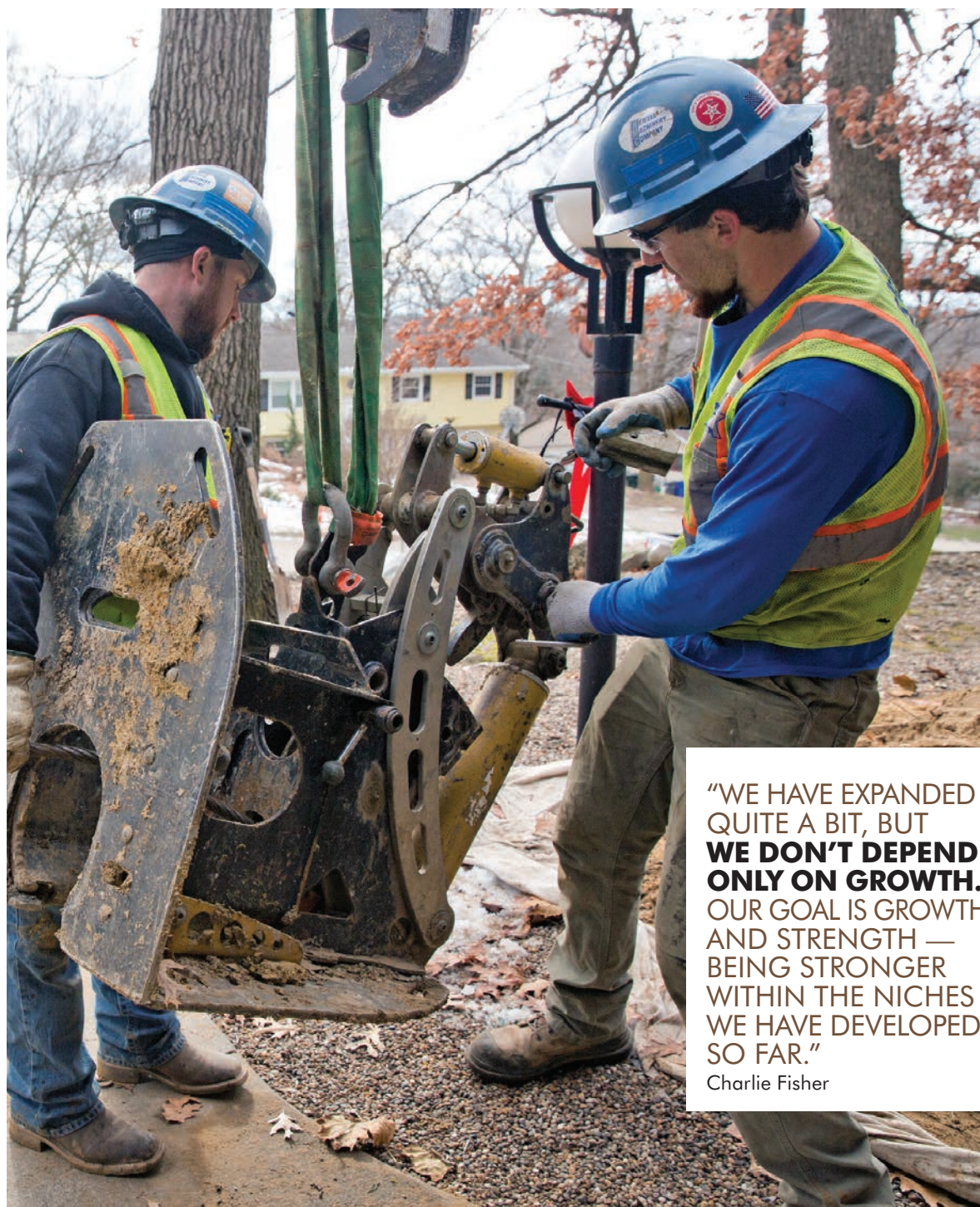
Kyle Jacobson (left) and Tucker Schroeder carry the PB30 pipe bursting machine (HammerHead Trenchless) to the job site pit.
