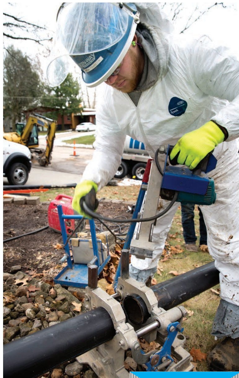
Mitch Fountain uses a Connectra Fusion Technologies system to join HDPE SDR17 pipe.
