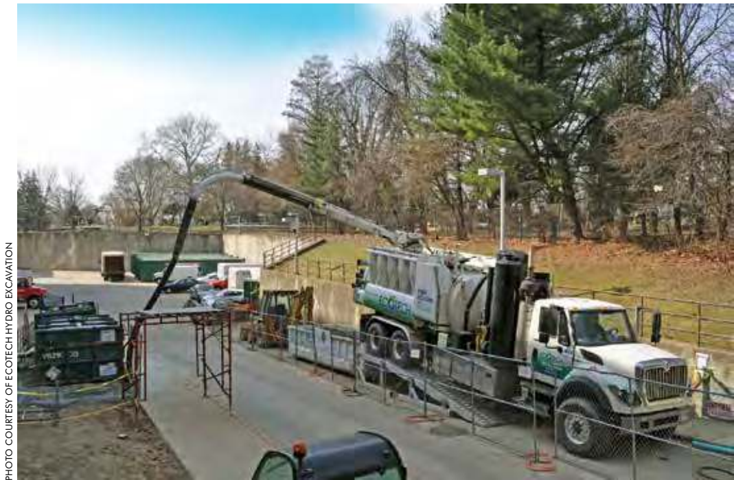
Pennsylvania-based Ecotech Hydro Excavation set up scaffolding to hold a hydroexcavator hose over the sidewalk to allow pedestrians to walk under for their safety on a job site at a hospital.
