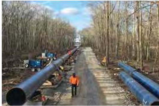
Crews weld together pipe segments in preparation of the underwater work after the HDD portion is completed. The pipes are then pulled into the lake and sunk where they are then attached to the segment that was installed using HDD.
