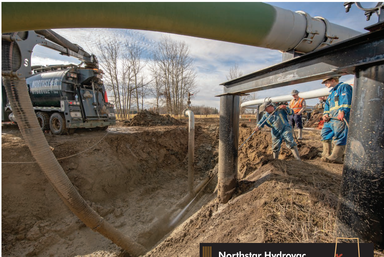
Stewart Caldwell, left, operator; Shaun Donavan, swamper; and Trevor Toyle, back, supervisor, expose a buried pipeline.
