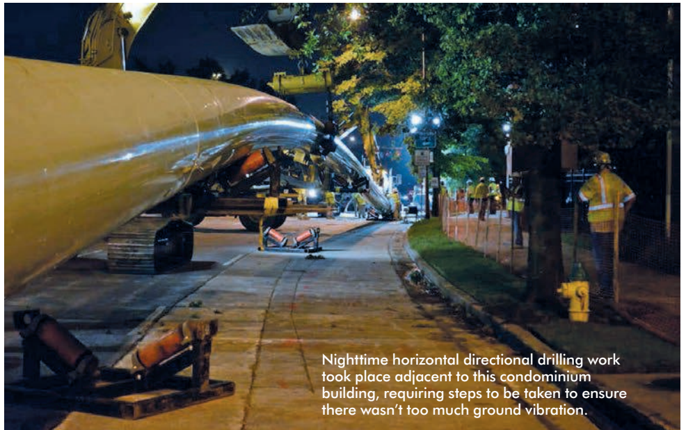
Pipe curvature and equipment support along major arterial roadway in downtown Norfolk, Virginia.
