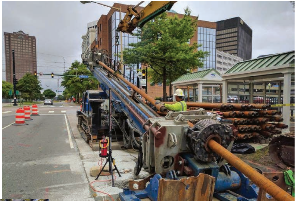
An American Augers DD-210 horizontal directional drill was used during the project in Norfolk, Virginia.
