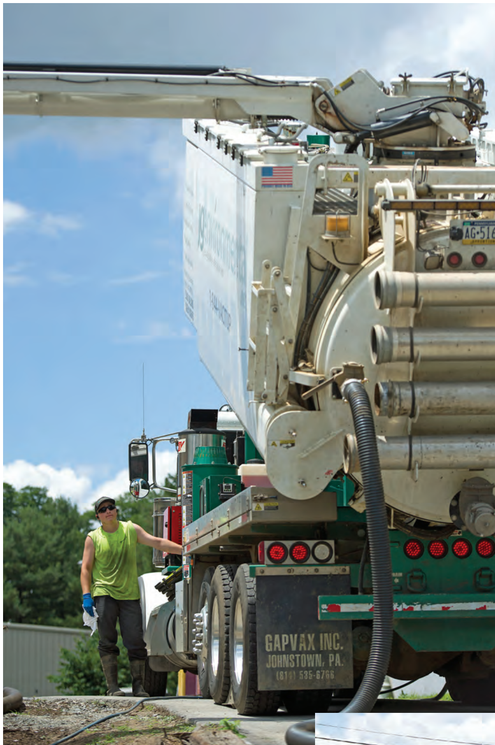
Brendan Perry, field service technician, drains the liquid from a GapVax hydroexcavator at a job site in Columbia, Pennsylvania.
