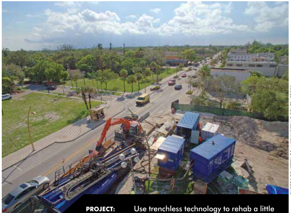
PHOTOS COURTESY OF MURPHY PIPELINE CONTRACTORS
