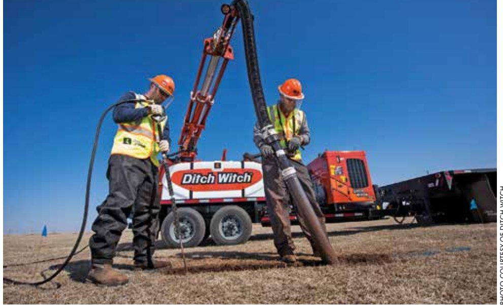
PHOTO COURTESY OF DITCH WITCH
