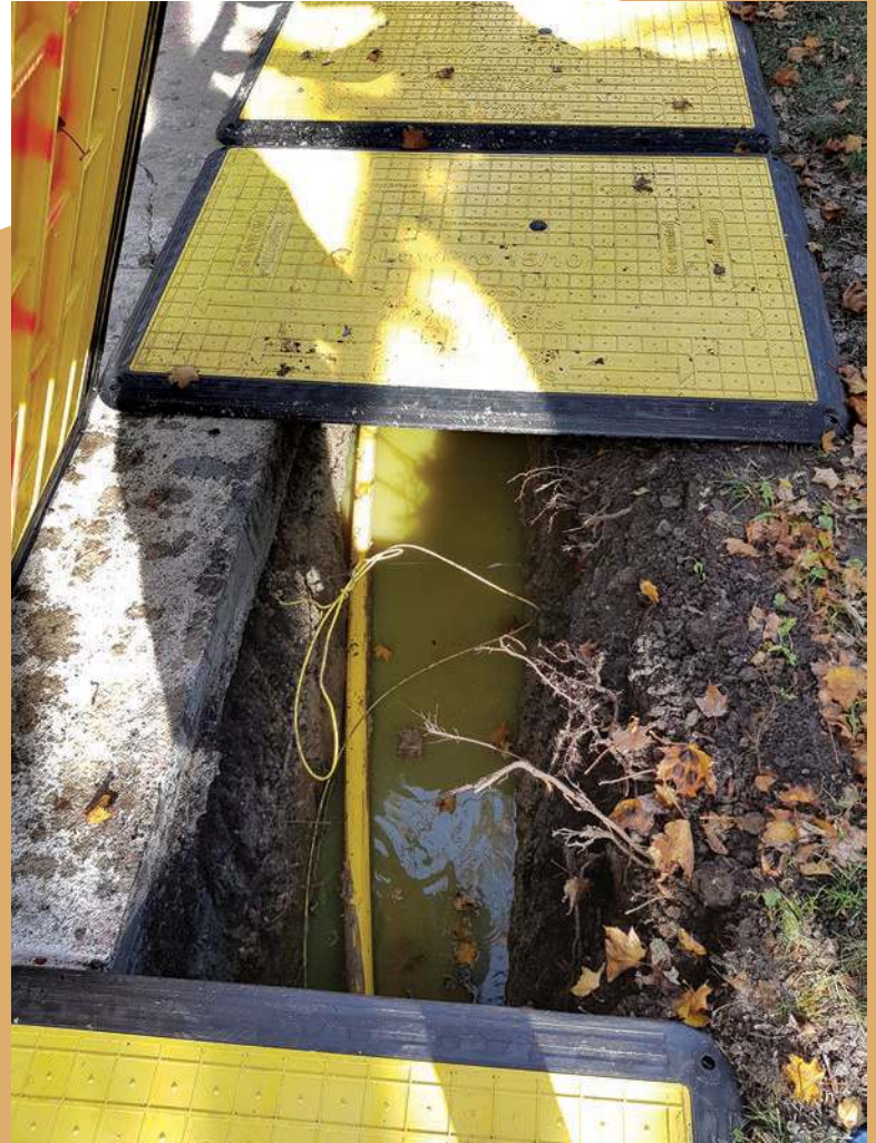
LowPro 15/10 trench cover system from Oxford Plastics
