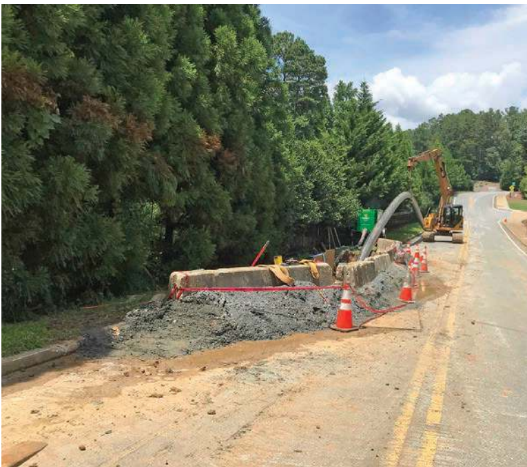
Approximately 2,200 linear feet of the 10-inch sewer on Kennesaw State University's campus was upsized through static pipe bursting.
