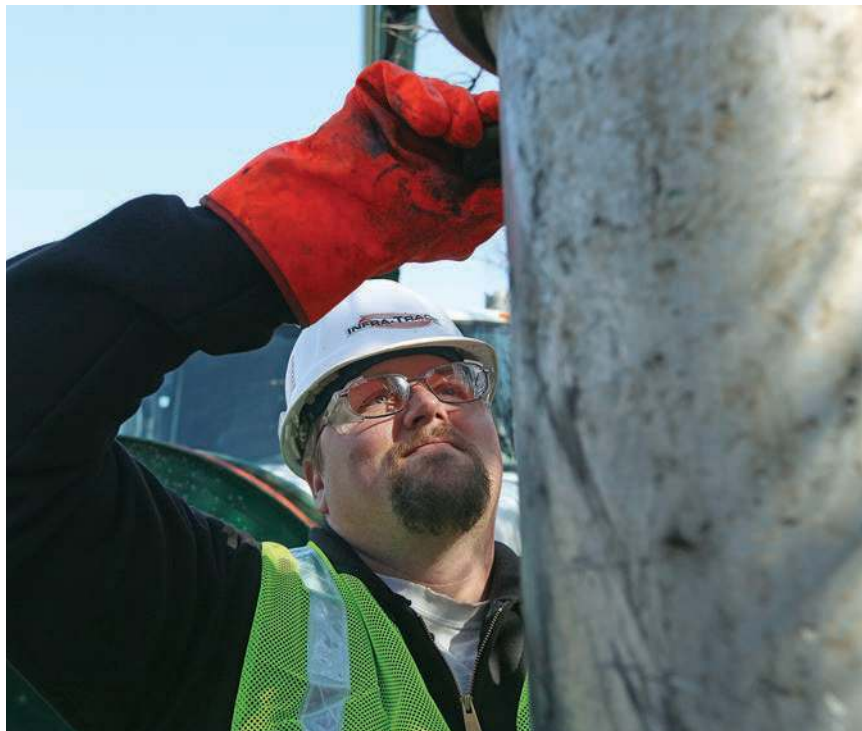
Nicholas Sees, Infra-Track lead service technician, attaches a vacuum tube to a Vac-Con truck on a job site near Canton, South Dakota.
