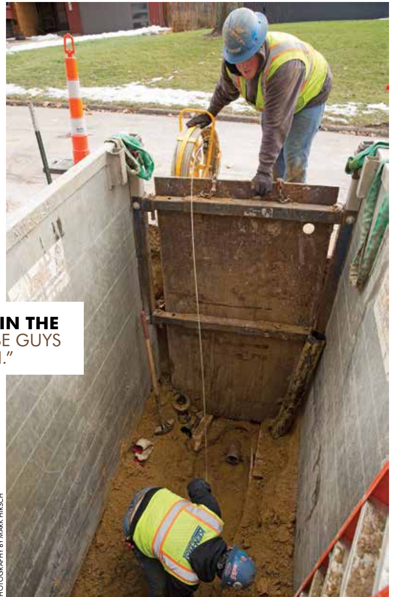
Crews from Ken-way Excavating use a trench box on a job site during a pipe bursting job.
