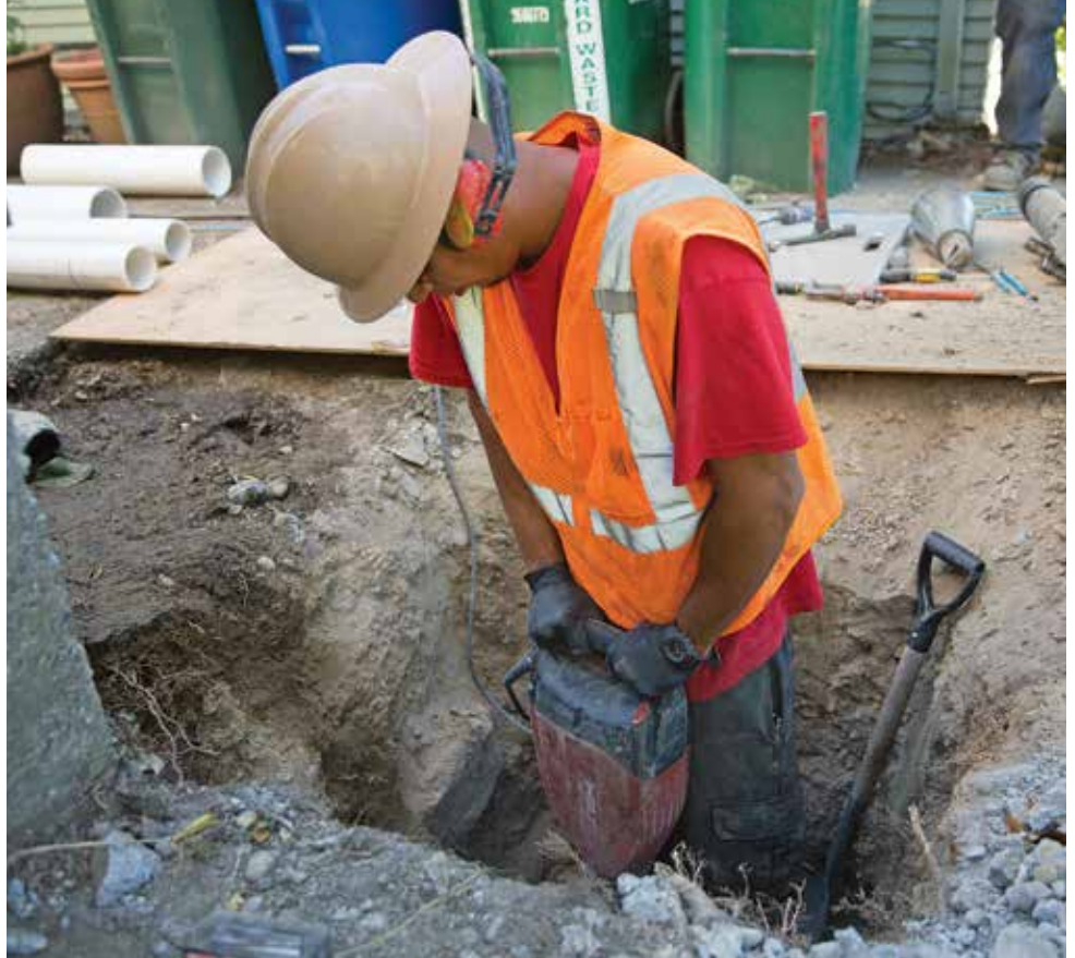
Technician Dan Woolcott digs an entry pit for a pipe bursting job at a home near Seattle.
