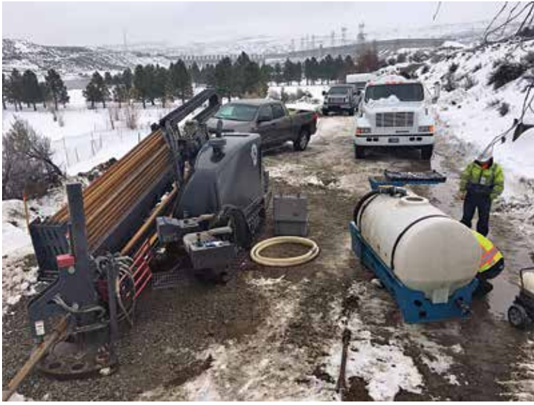
Allied Plumbing and Pumps staff use a horizontal directional drill on a job site in the winter on a line installation.
