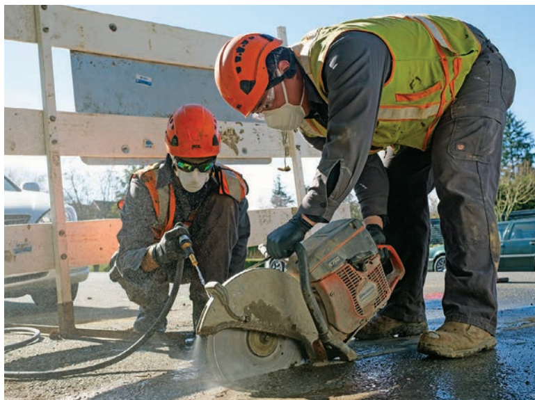
Chong, right, uses a Husqvarna K 760 power cutter to carve through asphalt as Dylan Leshner, apprentice, applies water while replacing a sewer line.
