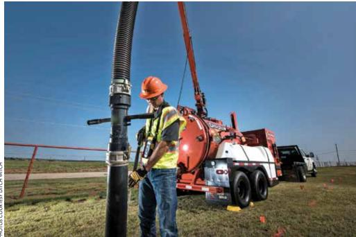
Vacuum excavation is becoming one of the go-to methods for utility locating and avoiding damage to underground utilities.
