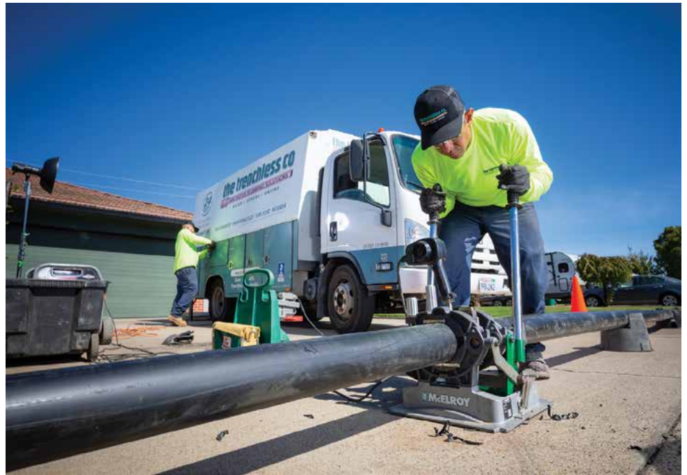
A crew from The Trenchless Co., based in Northern California uses McElroy pipe fusion equipment on a pipe bursting job. It is important for crews to understand how each piece of equipment works when on the job.
