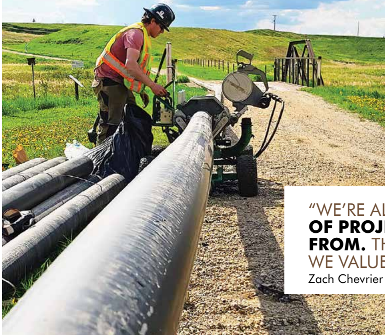
Zach Chevrier uses a McElroy pipe fusion machine to piece together pipe portions on a job site in western Canada.
