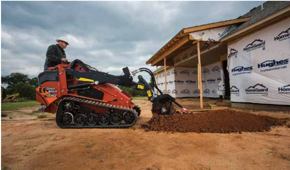
PHOTO COURTESY DITCH WITCH
