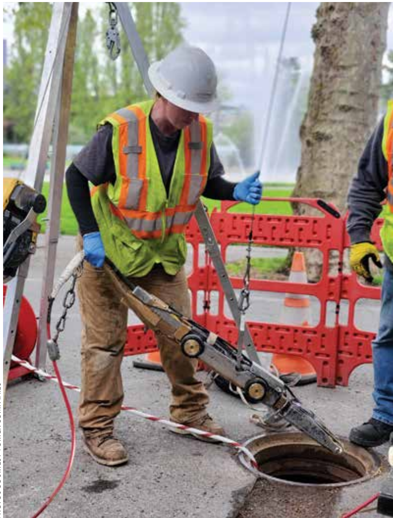
Vortex Companies' versatile Schwalm robots provide fast and efficient grinding, cutting, chiseling and cleaning capabilities for pipes 8 to 24 inches in diameter, as well as easy lateral reinstatements and point repairs.
