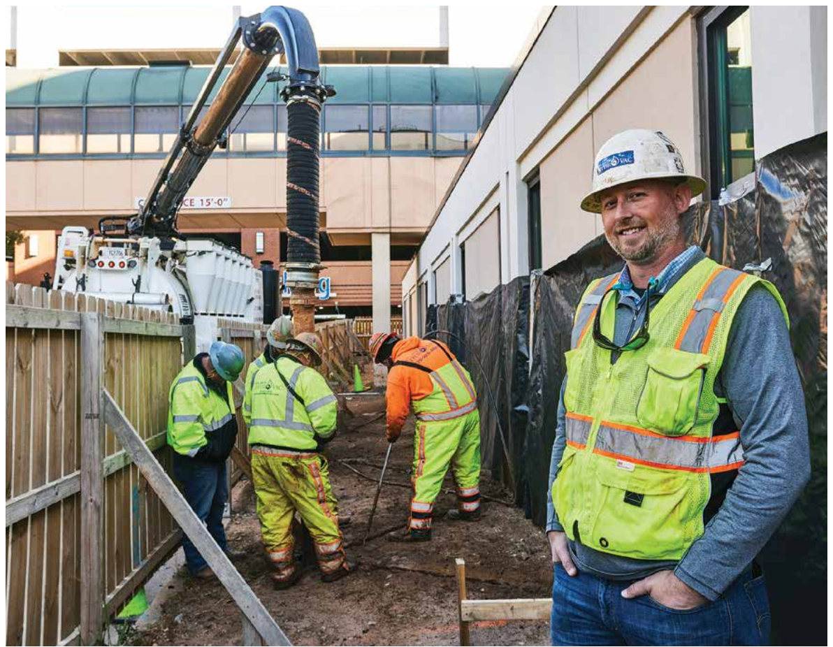
Atlanta Hydrovac general manager Greg Dubin (right) stands nearby a crew potholing for utilities using one of the company's GapVax HX56 units. Dubin joined the company a year after it was started.
