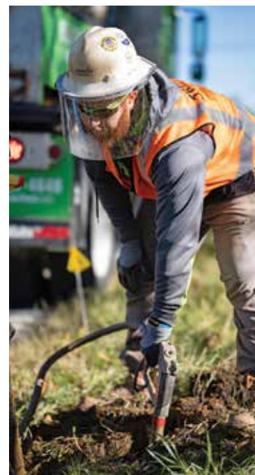
Jordan Cohen reaches down with the digging lance into the hole being dug to look for utilities along the roadway. The company uses a Vactor Paradigm and a Vactor 2100 for vacuum excavation work.
