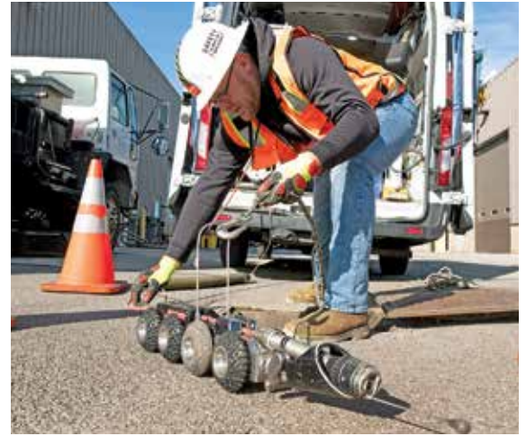
Adam Geer, a field service tech, prepares to use a lateral launch crawler (Envirosight) on the campus of the University of Toledo.
