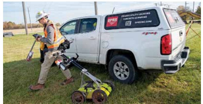
GPRS project managers switch between ground-penetrating radar systems while on a job sites to locate utilities. The company uses Chevrolet pickup trucks to service all 50 states.
