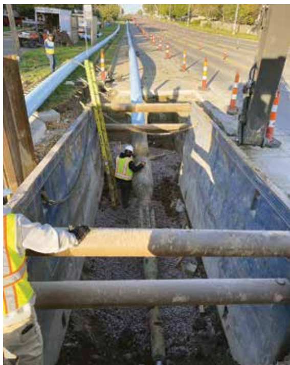
ABOVE: The Siteworks crew replaced the existing mains with 16- and 20-inch fusible PVC. LEFT: The project included pipe bursting 2,000 feet of 16-inch cast iron main and 2,200 feet of 20-inch ductile iron main. Crews used a 1900G Grundoburst static pipe bursting system.
