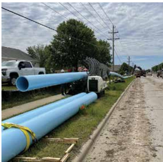
ABOVE: The Siteworks crew replaced the existing mains with 16- and 20-inch fusible PVC. LEFT: The project included pipe bursting 2,000 feet of 16-inch cast iron main and 2,200 feet of 20-inch ductile iron main. Crews used a 1900G Grundoburst static pipe bursting system.
