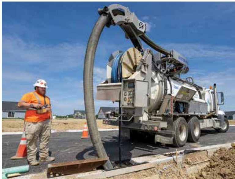
Heavy Equipment Operator David Beeman Fonseca uses a KAISER PREMIER EcoCycler to jet a storm line in a neighborhood for a post-clean inspection.
