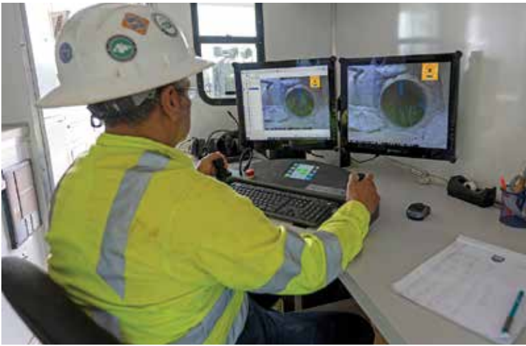
PACP Camera Operator Freddy Garcia operates a Rapidview IBAK HD Mainline System televising a neighborhood for a post-clean inspection.
