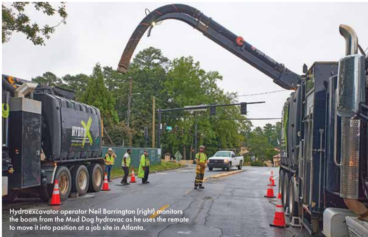
The digging wand effectively exposes utilities using high-pressure water.
