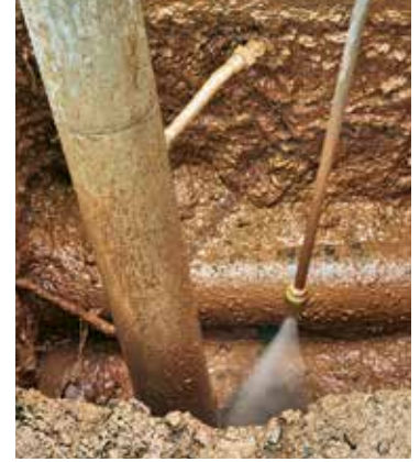
The digging wand effectively exposes utilities using high-pressure water.
