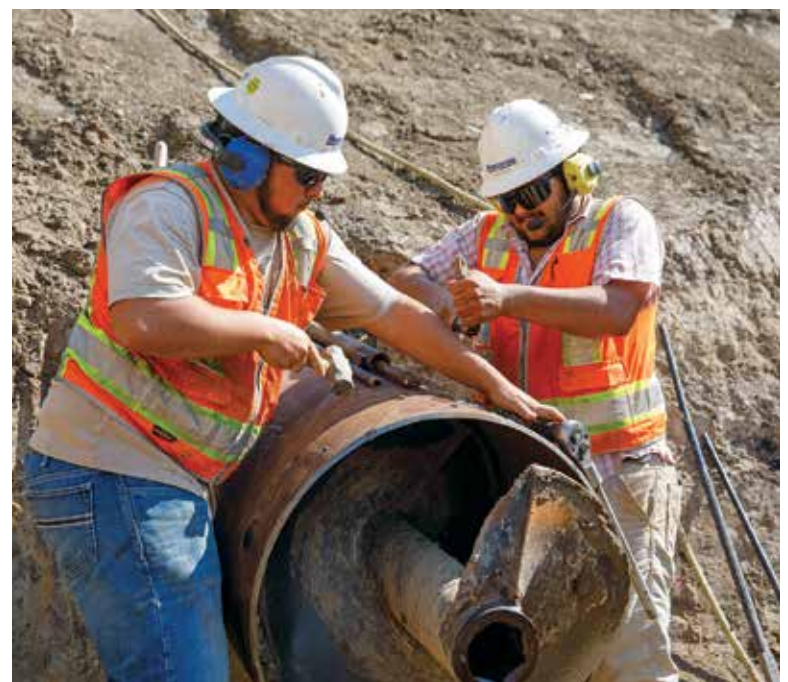
Martinez (left) and Rodriguez fit piping to a culvert extension.
