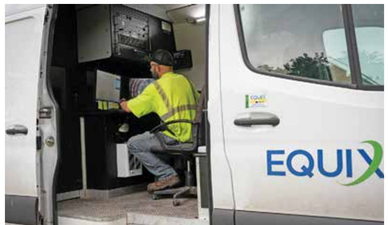
The company performs pre- and post-construction inspections to map existing cross bores and locations of laterals. Here Albanese works in the CCTV inspection van (CUES).
